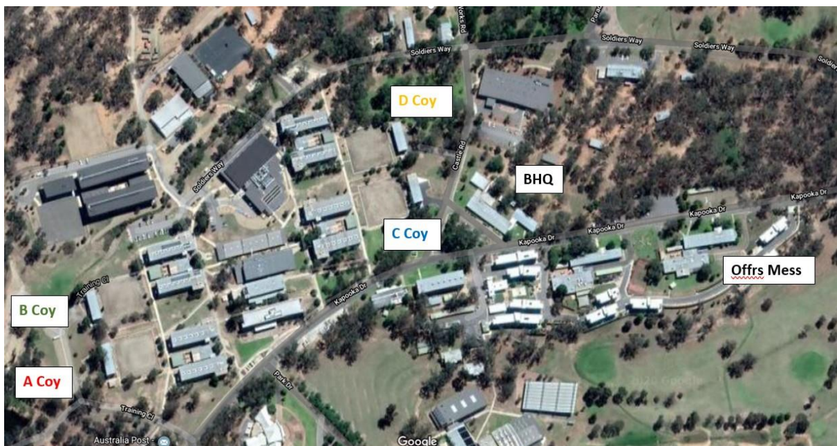
1 RTB Kapooka with 1969 buildings marked
